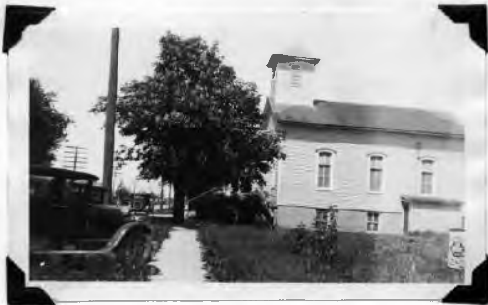
Church Building repaired with shortened steeple.
